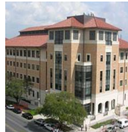
Biomedical Engineering Building (BME)
